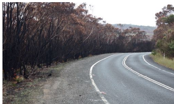
Fire-affected areas along a section of Sir Bertram Stevens Drive.
